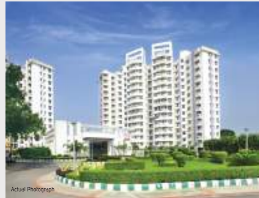
Eldeco Eternia Sitapur Road, Lucknow
